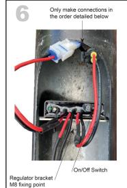
Moving to the column base, fix the regulator plate in the base with the M8 hex socket set screw and nuts supplied.
