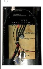
Moving to the column base, fix the regulator board in the base with the 8mm hex screw supplied.
