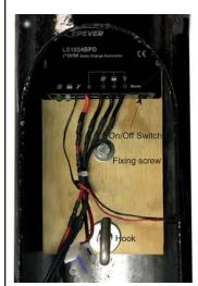
Moving to the column base, fix the regulator board in the base with the 8mm hex screw supplied.
