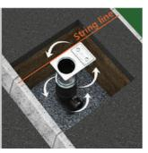
**6**Using levelling pole, check vertical alignment.
