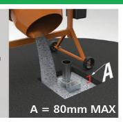
Insert socket, orientate top and bottom to suit. Set finished level with string line.
